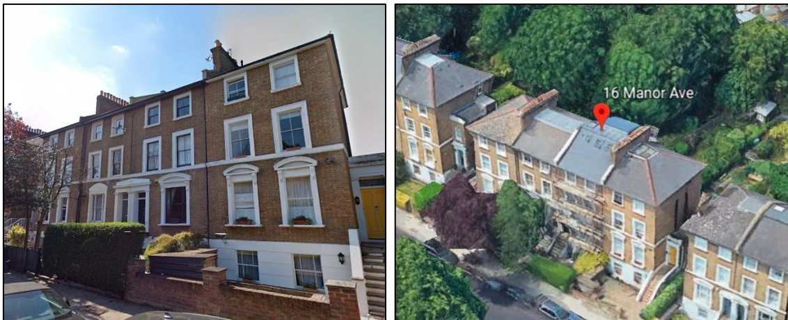
Photo 2. Front roof slope of No.17 Manor Avenue
