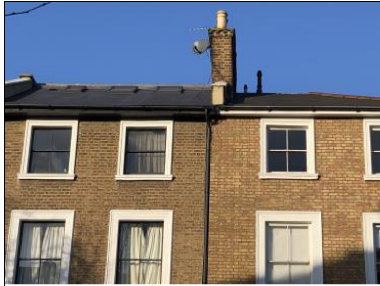
Photo 1. Front roof slope of No.16 Manor Avenue
